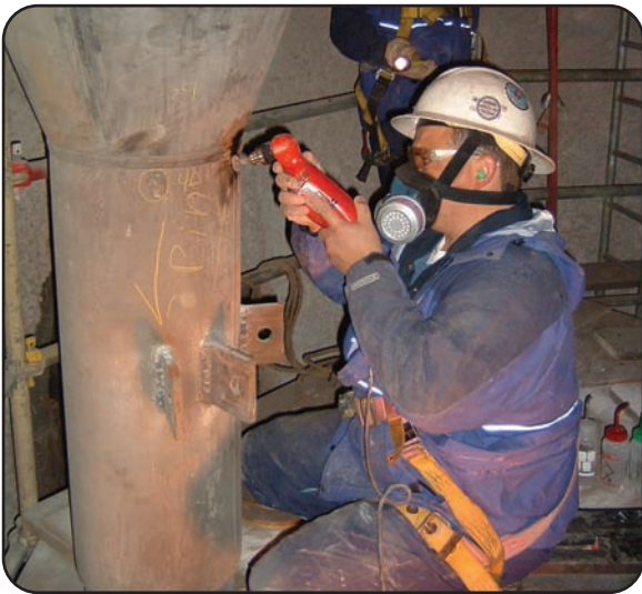
In-situ surface preparation
