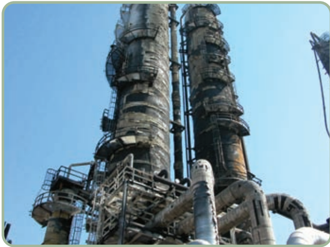
(above, below) Vessel Fire Damage Assessment
