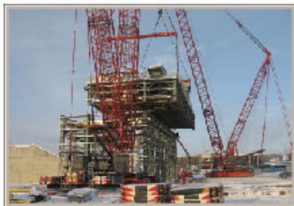
Hoisting and Placement of Roof Structure
