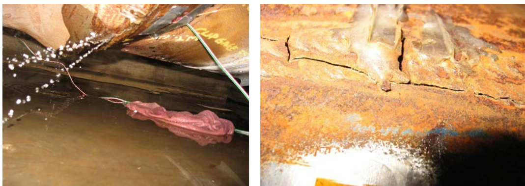
Figure 10. Leak during burst test after reaching 1,434 psi (photograph taken at approximately 15 psi).
