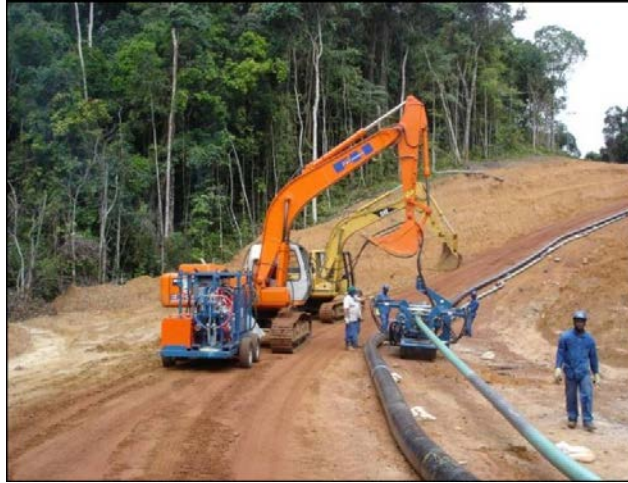
Figure 1. Onshore installations using the interference fit connection process
