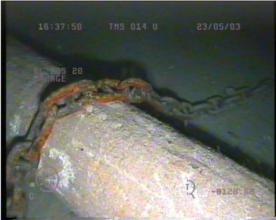
Figure 8 – Image of damaged subsea pipeline via ROV camera [16]
