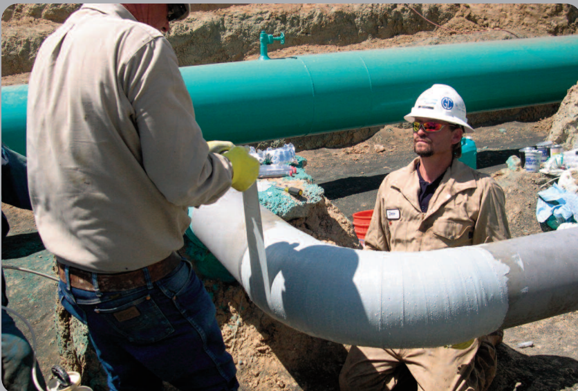
Figure 1 Composite field repairs being completed by Armor Plate, Inc.
