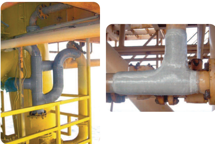
Figure 3 Illustration of challenging field applications of composite repairs. Images provided by Armor Plate, Inc.
